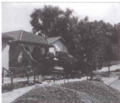
Drainage work underway.
