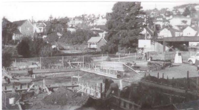
The convent foundation being laid, February 11, 1949.
