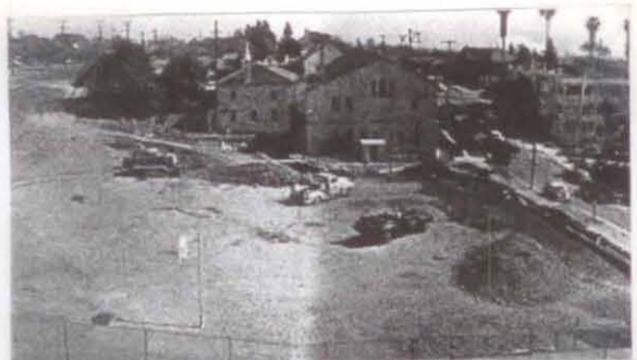
Excavation of the "wasteland" underway, April 1954.
